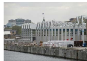
Figure 104. Chantier du Village de la Construction
